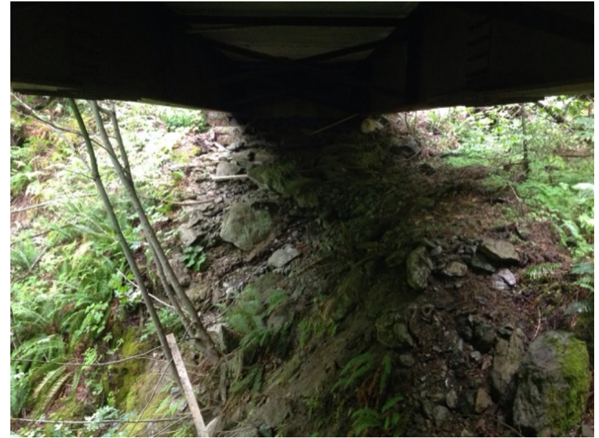
Right Bank Abutment when facing downstream
