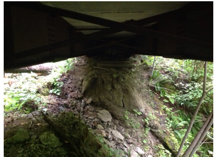
Left Bank Abutment when facing downstream
